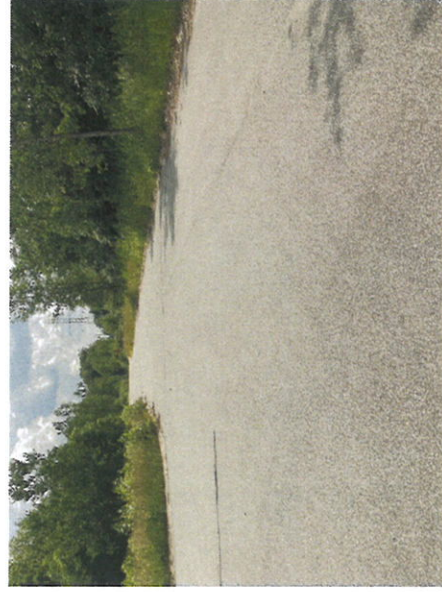
Phase 1 pavement alligator cracks and previous repairs (Levanno Drive shown)
