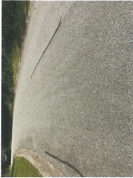
Phase 1 pavement cracks (Verdano Terrace and Levanno Dr shown)
