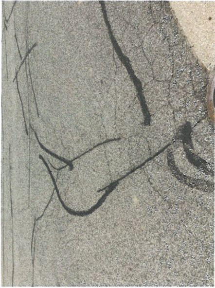
Phase 1 pavement cracks (Verdano Terrace and Levanno Dr shown)
