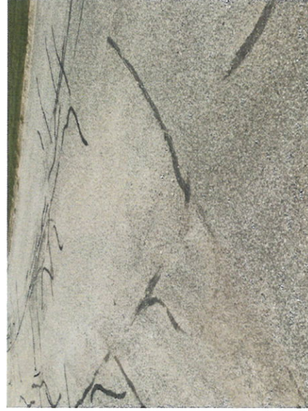
Phase 1 pavement cracks – note previous repairs (Levanno Drive shown)
