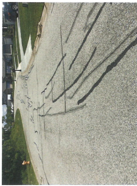
Phase 1 pavement cracks (Verdano Terrace near clubhouse shown)
