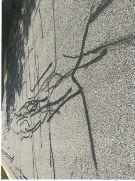
Phase 1 pavement cracks – note previous repairs (Levanno Drive shown)
