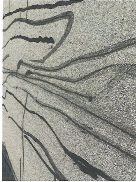
Phase 1 pavement cracks and previous repairs (Morena Terrace shown)
