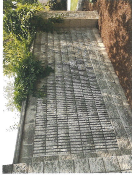
Masonry perimeter wall overview
