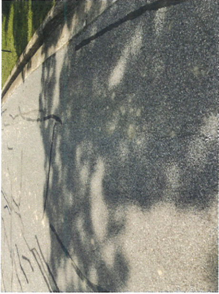
Phase 1 pavement cracks and previous repairs (Morena Terrace shown)
