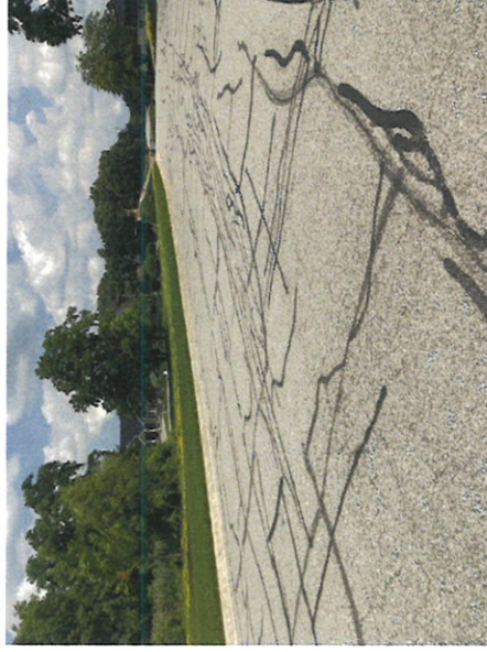
Phase 1 pavement alligator cracks and previous repairs (Levanno Drive shown)
